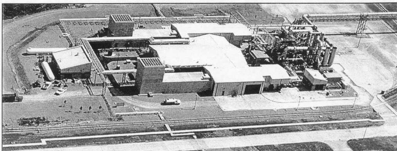
SL2 and SL3 were constructed at AEDC, Tullahoma, TN, to perform the type of testing that was previously accomplished in 1W and 2W at NAWCAD-TRN
